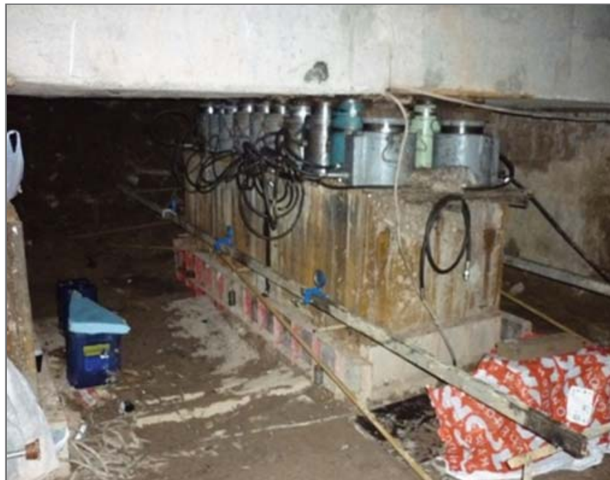
Fig. 2. A set of 22 synchronized jacks DGO-200 with auto support station on the head of the tested barrette pile. (photo by E.A. Parfenov).
